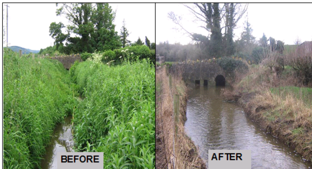
Figure 5-4: Dredged River (Segment 19) showing the before and after Photos
