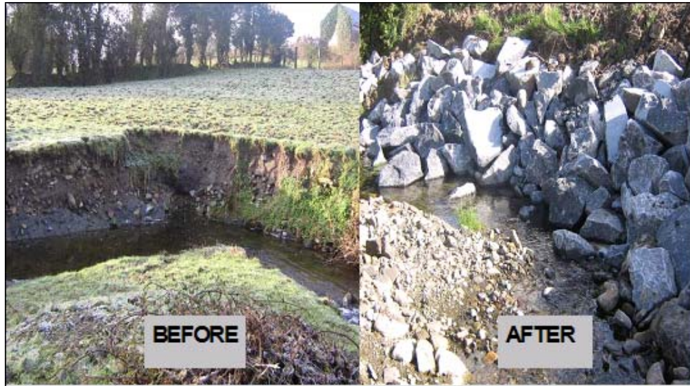
Figure 5-5: Dredged River (Segment 30) showing a Deposit of Boulders on one Bend to Support a New Road along the River Bank
